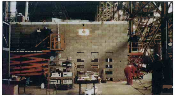
BRE/FRS Full-Scale Test Rig (side view)
