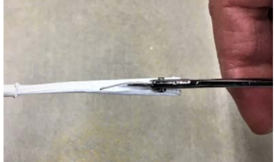
Cut binder tape lengthwise with a small scissors
