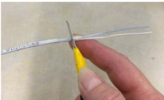
Score/crack jacket for solder sleeve
